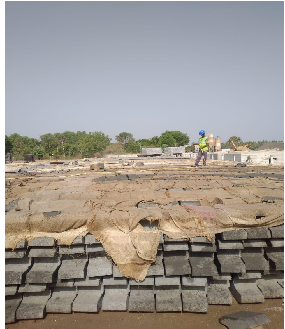
RE block casting and curing at camp casting yard
