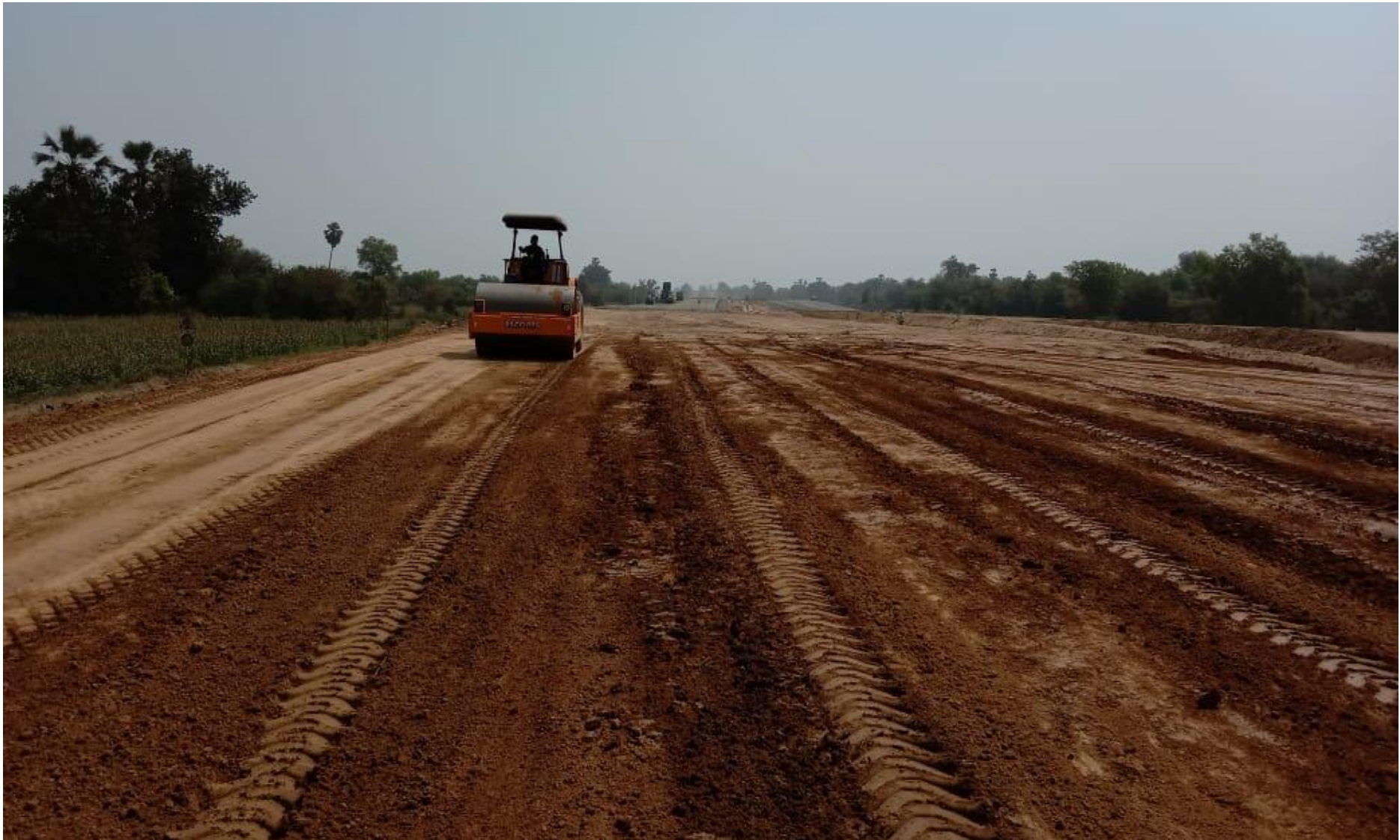
Embankment Layer in progress
