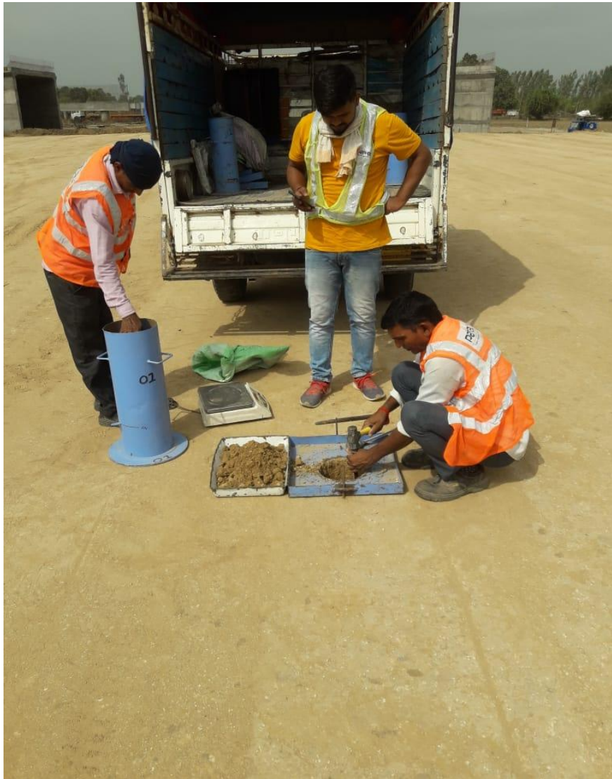
FDD checking at Ch. 351+250
