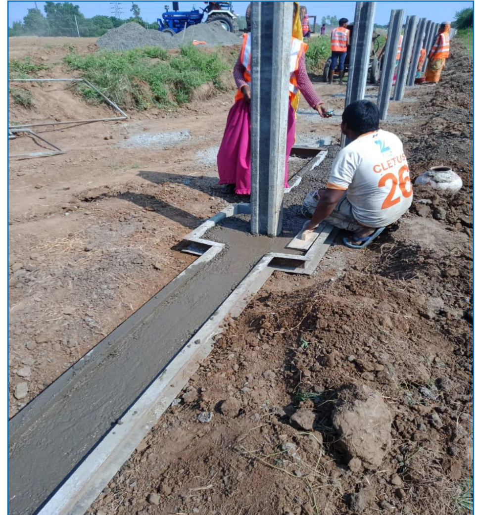
Fixing of Boundary wall work in progress at ch. 357+000 to 357+200
