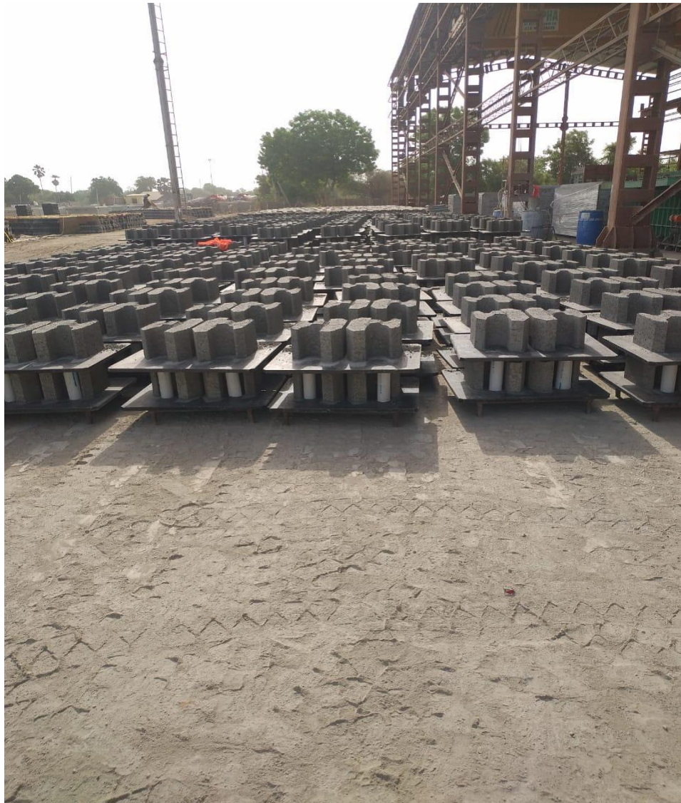
RE block casting and curing at camp casting yard
