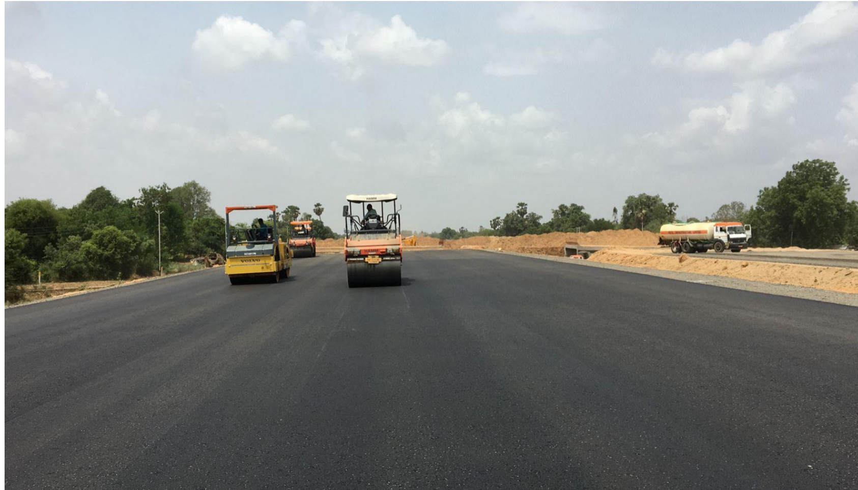
DBM-1st Rolling In Progress
