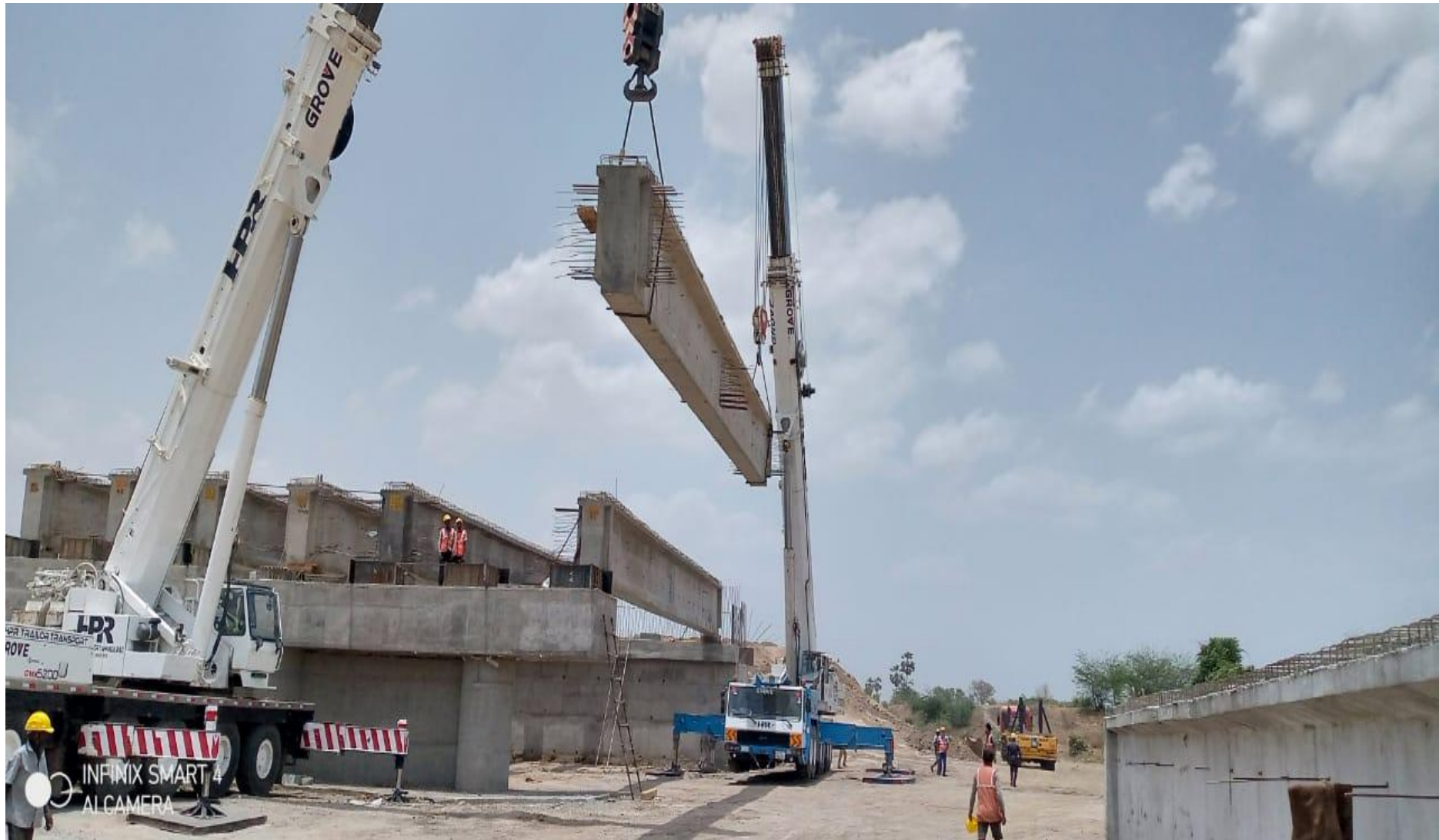
Girder launching at Major Bridge Ch-359+936
